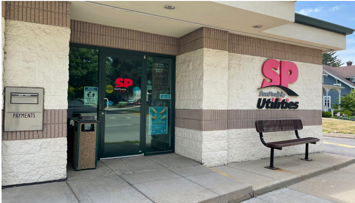
(Photo: Sun Prairie Utilities Main St. operations facility.)
